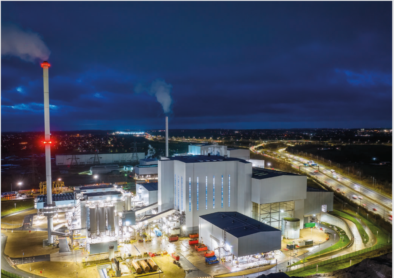
enfinium's Ferrybridge facility in West Yorkshire is home to the largest single waste-to-energy site in the UK
